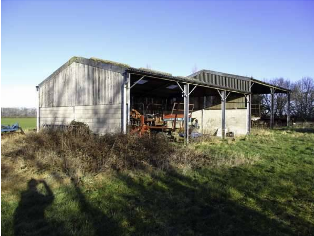
Photograph 6: Farm Building to the northeast corner of Field 6
